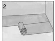
Always use an underlayment padding above the vapor barrier and below the laminate flooring planks. If pad is pre-attached, no additional underlayment should be used.
